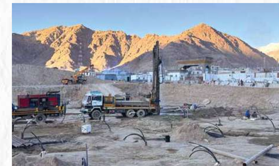
Application of Geo Thermal Energy for carbon neutral Leh Airport.
