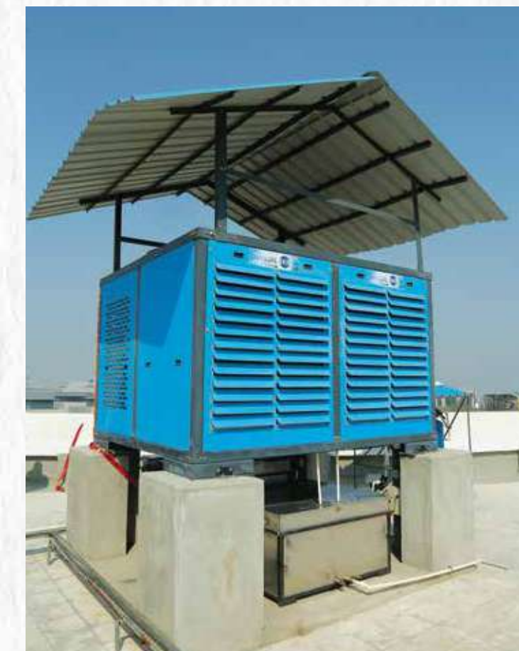
2000 LPD Atmospheric Water Generator (AWG) unit, powered by solar energy, installed at EIL R&D Centre, Gurugram (Vayujal Technologies Pvt. Ltd.).
