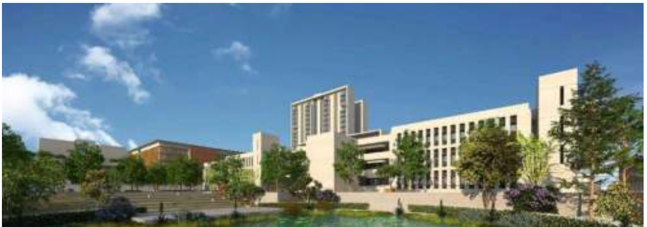
RBI Green Field Data Centre in Bhubaneswar
