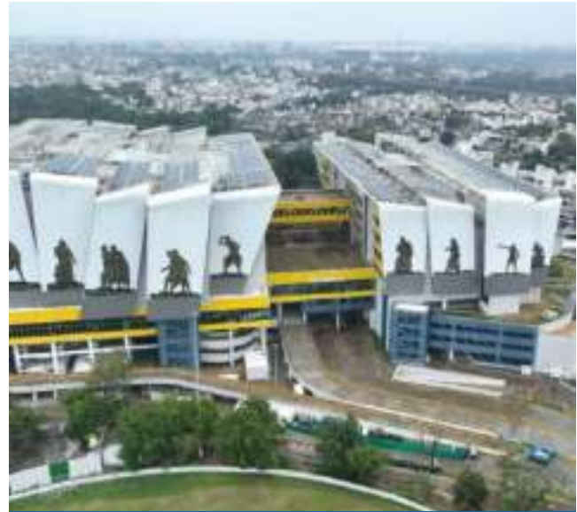
Completion of Sabarmati High-Speed Rail Terminal in Ahmedabad, Gujarat
