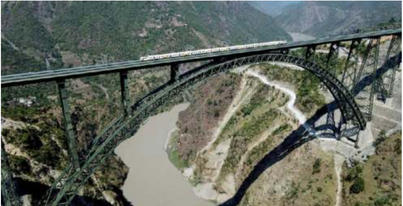
Chenab Bridge High Speed Test Run
