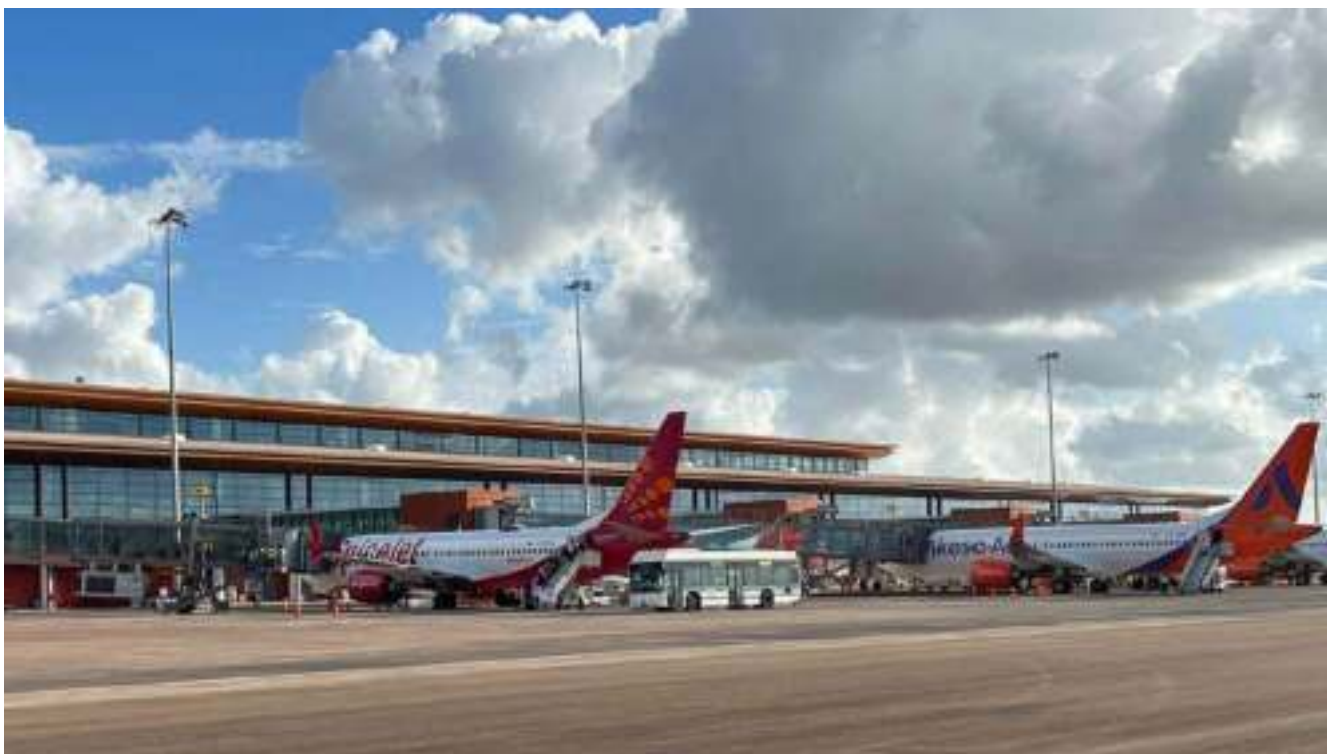
Passenger Terminal Building at Goa International Airport
