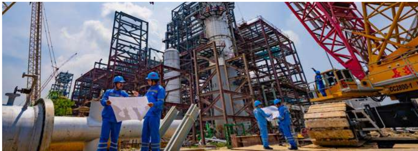
Panipat Refinery Expansion Project (P-25)
