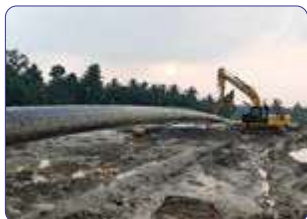
Dobhi-Durgapur-Haldia Pipeline Project
