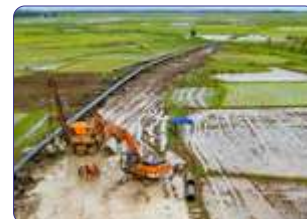
Upgradation of facilities for Numaligarh-Siliguri Pipeline
