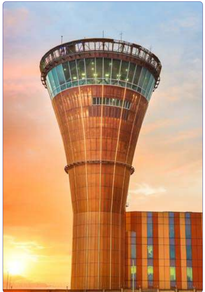
Air Traffic Control Tower at Mopa International Airport, Goa
