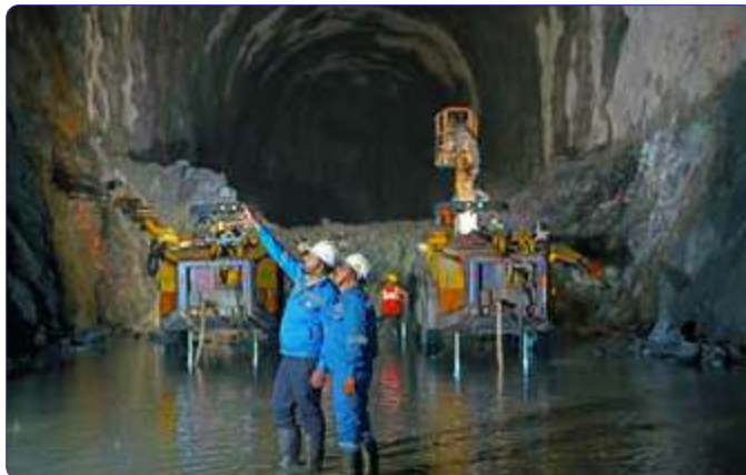
LPG Cavern Project, Mangalore
