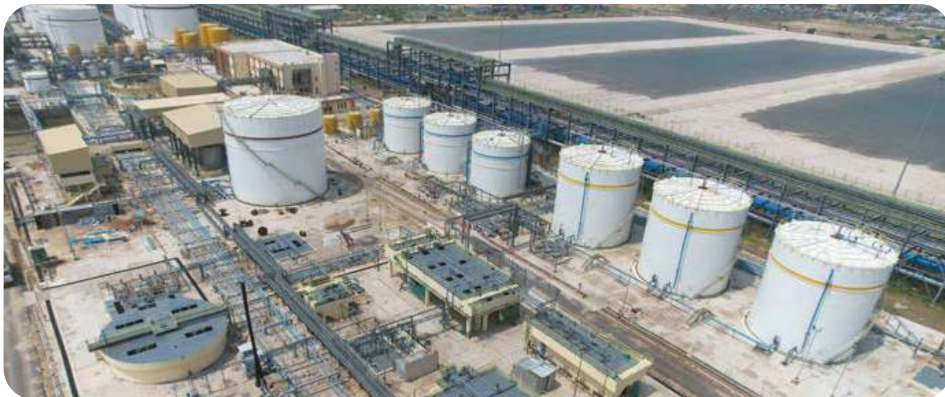
Effluent Treatment Plant (ETP) at Rajasthan Refinery Project
