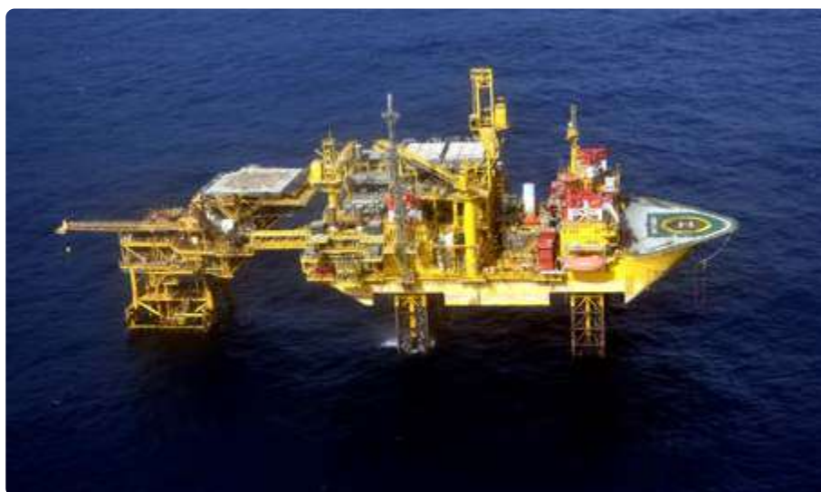
Sagar Samrat- a transformed Mobile Offshore Production Unit (MOPU)
