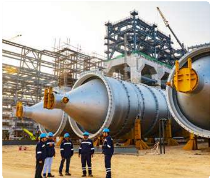
Rajasthan Refinery project
