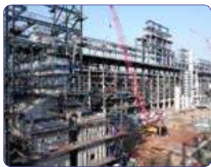
Setting up of PPU Project at Numaligarh Refinery
