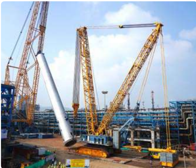
Erection of the world's heaviest LC-Max Reactor in the RUF Unit of VRMP, Visakh Refinery
