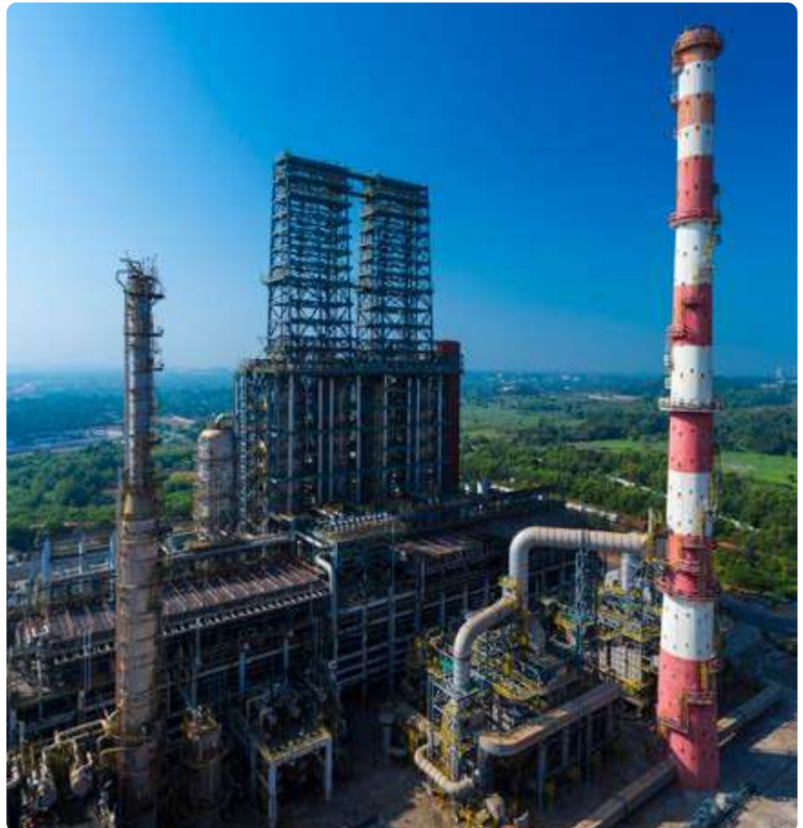
Delayed Coker Unit (DCU) at Mangalore Refinery
