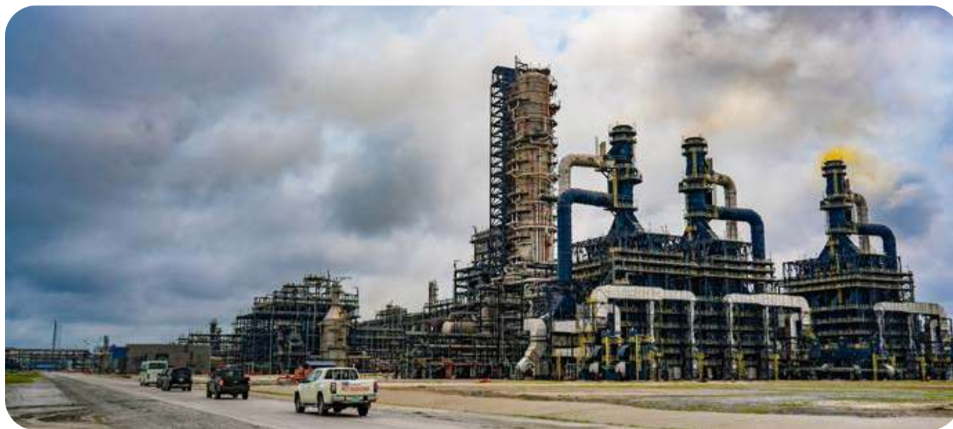
Dangote Refinery Project, Nigeria
