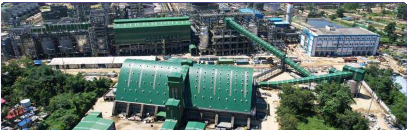
Assam Bio Refinery Project in Numaligarh
