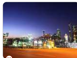
Ethylene Cracker and U&O for Bina Petrochemical & Refinery Expansion Project
