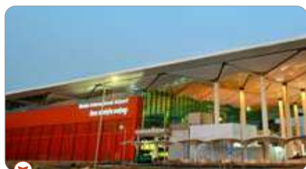
Greenfield Noida International Airport, Jewar, Uttar Pradesh
