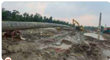
Dobhi-Durgapur-Haldia Pipeline Project
