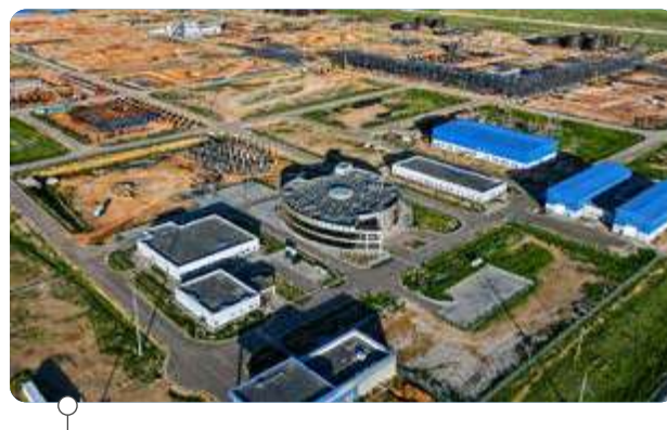
Crude Oil Refinery Project in Mongolia
