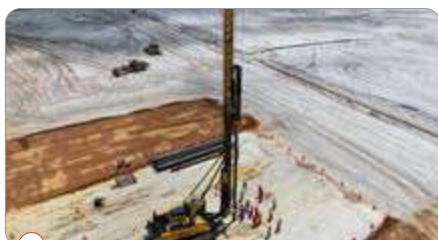
Guyana Integrated NGL Plant and 300 MW CCGT Power Plant Project
