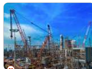
PPU and Revamp of PFCC Project at Kochi Refinery
