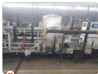
Replacement & Additional Installation of Compressors
