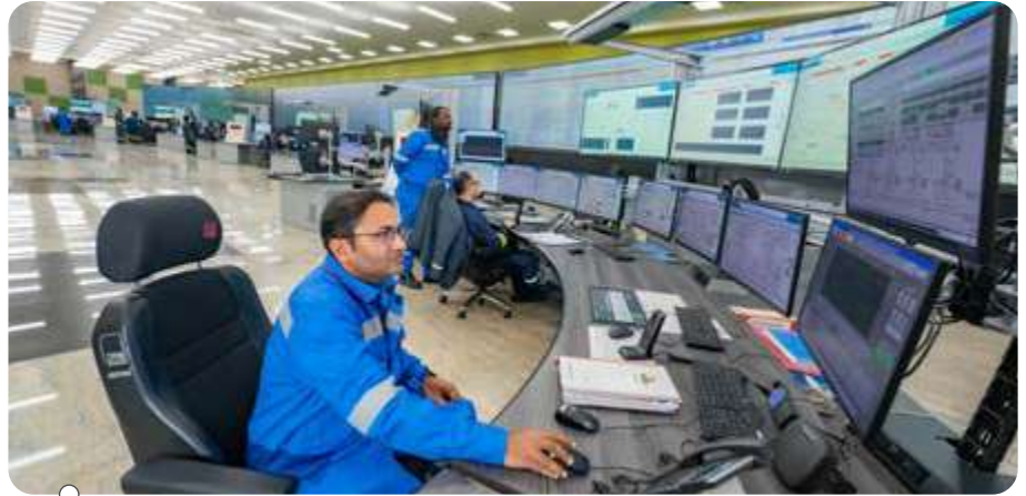
Main Control Room at Guru Gobind Singh Refinery, Bhatinda
