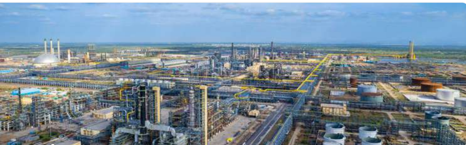
Rajasthan Refinery project, Barmer
