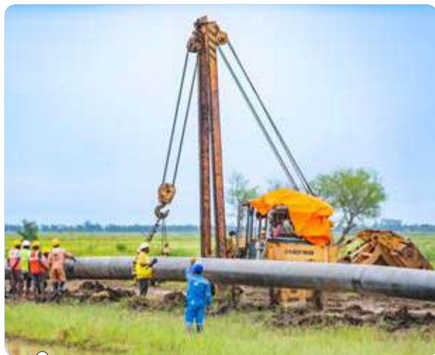
Paradip-Numaligarh Crude Pipeline (PNCPL) project
