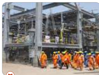
Revamping of SV Stations, Gas Terminal & Kribhco Terminal at Hazira Plant
