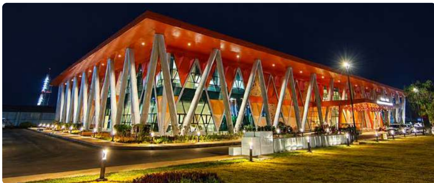
Management Development Facility at ATI, Goa
