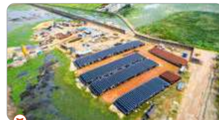
Upgradation of facilities for Numaligarh-Siliguri Pipeline
