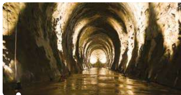
LPG Underground Storage Project, Mangalore
