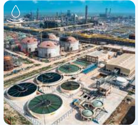
Water & Wastewater Management
