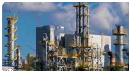
New Fertilizer Plant (Trains 3, 4, 5, &amp; 6) in Lekki Free Trade Zone- Nigeria
