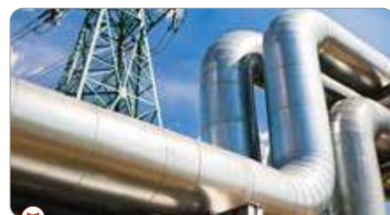
Capacity Expansion of Jamnagar-Loni Pipeline (JLPL) Project
