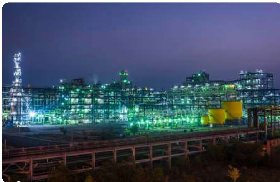
C 2 /C 3 Recovery Plant, Vijaypur (MP)
