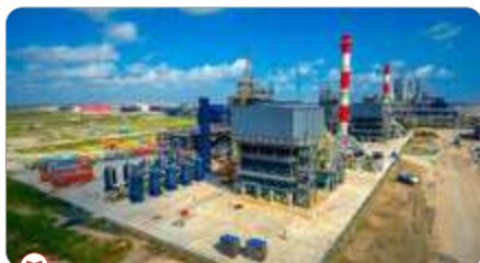
Expansion of Integrated Refinery cum Petrochemical Complex (Train 2)
