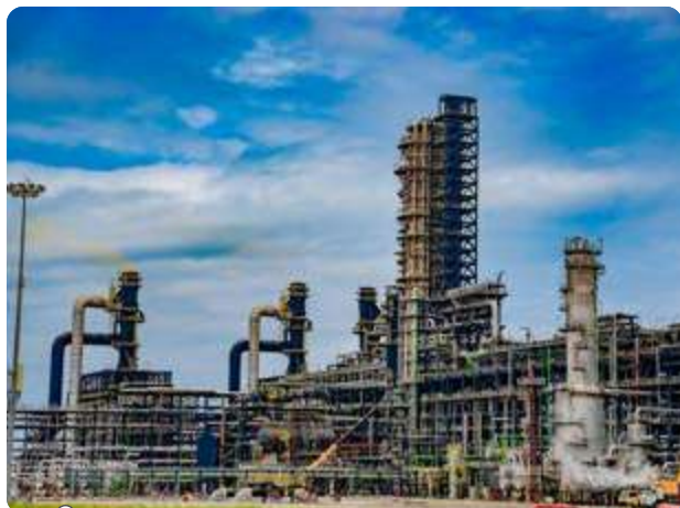
Dangote Refinery project, Nigeria
