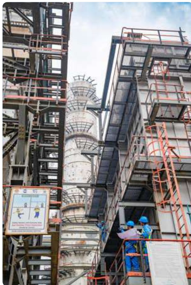
P-25, Panipat Refinery Expansion Project
