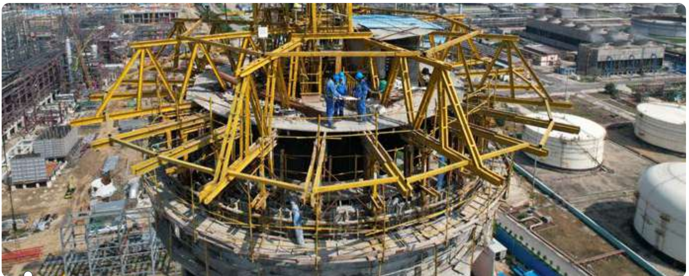
P-25, Panipat Refinery Expansion Project
