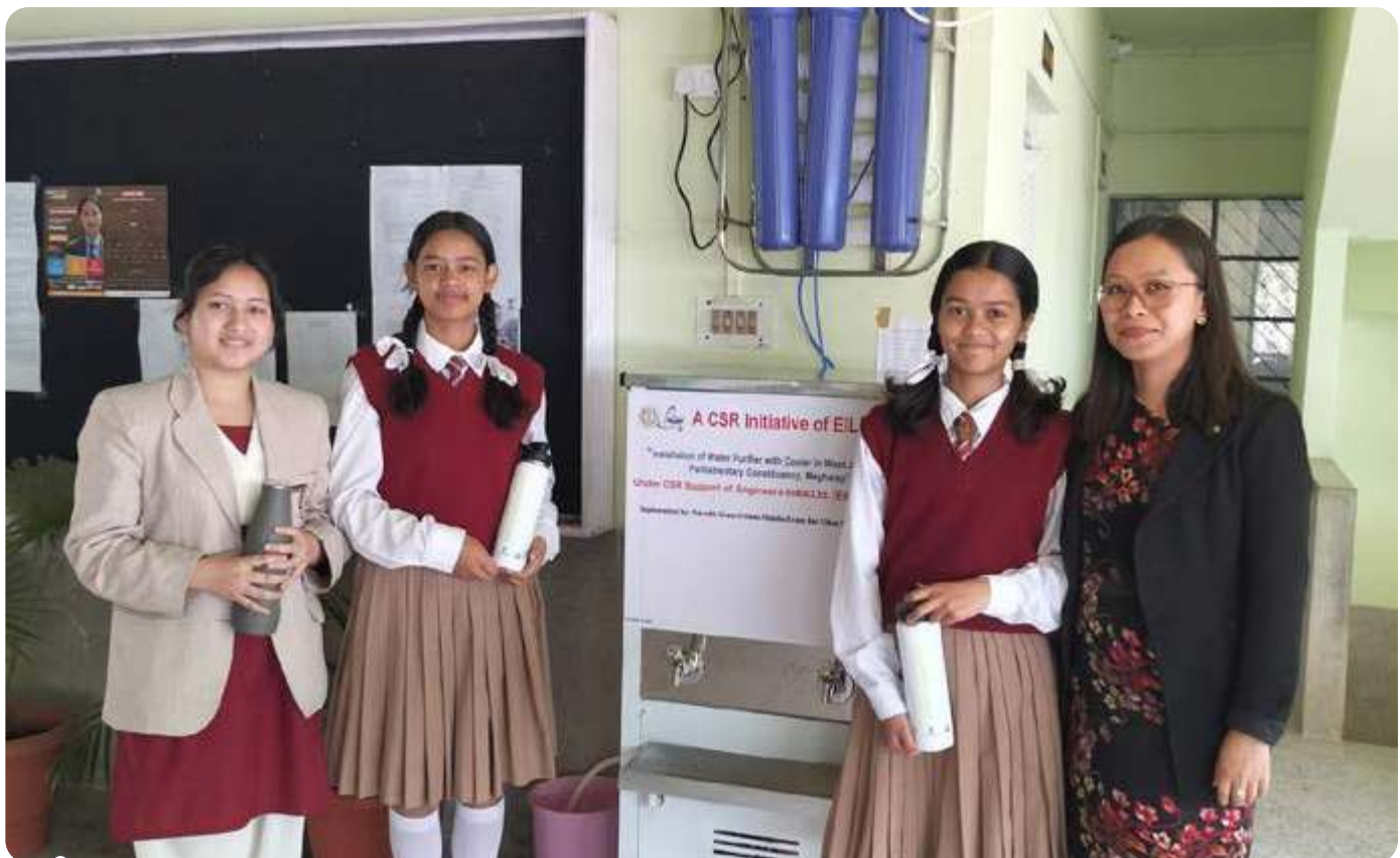
Installation of water purifiers for Govt. schools in aspirational district of West Jaintia Hills, Meghalaya
