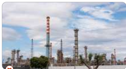
Aditya Aluminium Smelter Expansion Project at Lapanga
