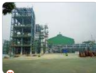
Setting up PPU at Numaligarh Refinery
