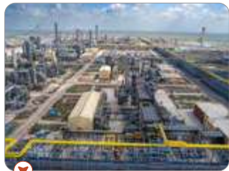
Rajasthan Refinery Project (HRRL)
