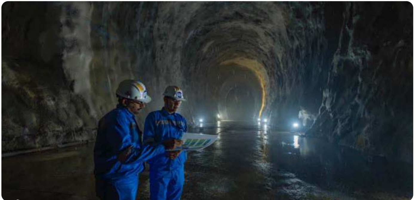
LPG Cavern Project, Mangalore
