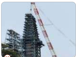
Delayed Coker Unit (DCU) Revamp Project
