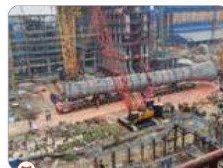
Coker-B Revamp Project
