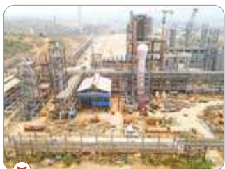
500 KTPA Petrochemical Project (PDH/PP)
