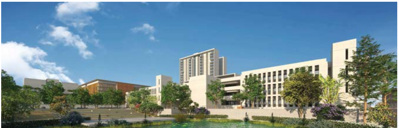
RBI Green Field Data Centre in Bhubaneswar
