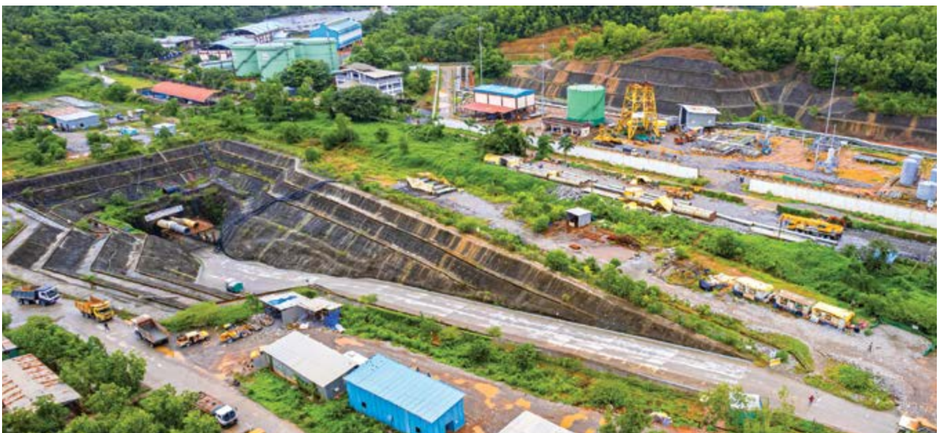
LPG cavern at Mangalore, Karnataka
