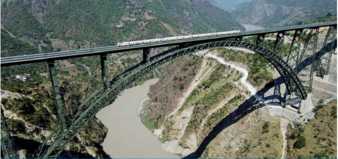
Chenab Bridge High Speed Test Run
