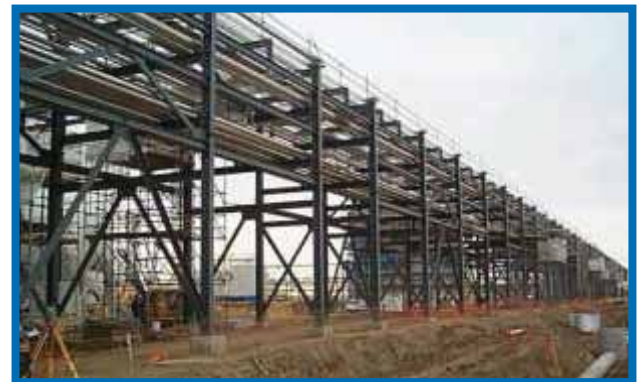
Fig. 13: Pipe rack Structure
